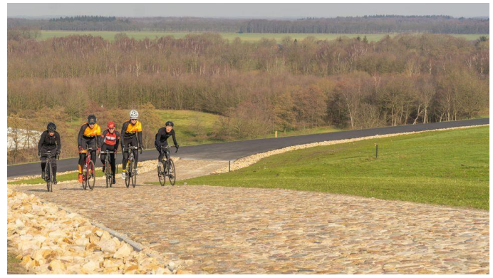
Col du VAM Former landfill: source www.drenthe.nl
